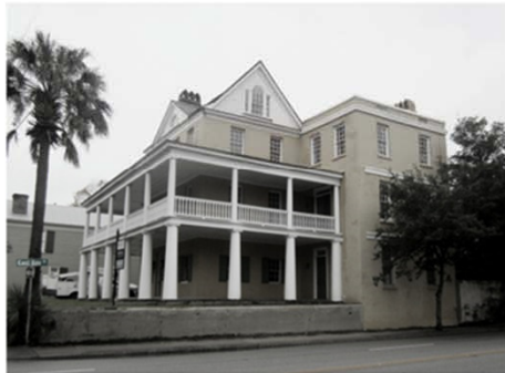
The Presqu'ile House, completed in 1808, at the corner of the project block is a good example of the grander residential structures along East Bay Street.
