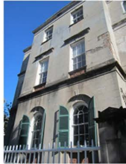
Windows nested within masonry recesses on a William Jay design on Meeting Street.
